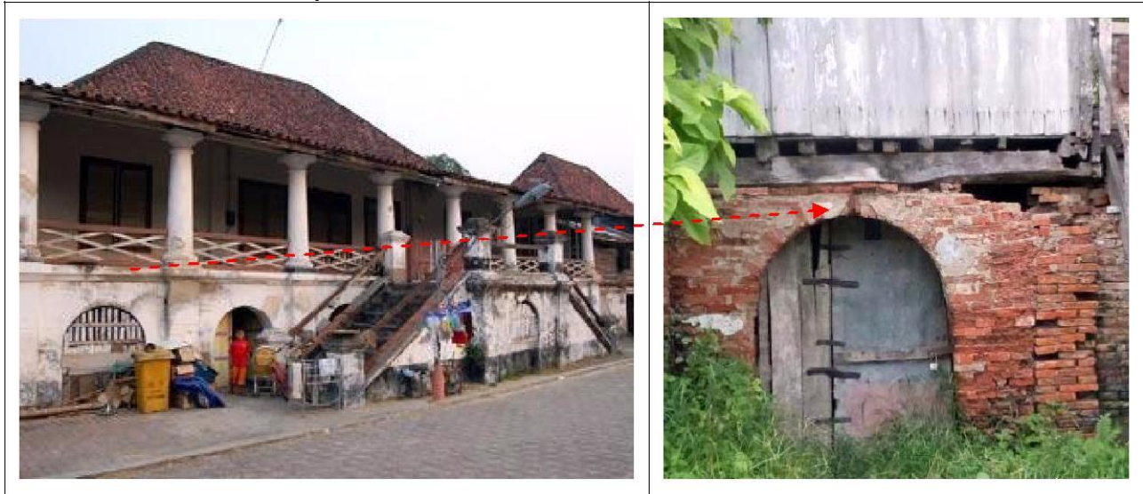
Figure 10. Tiled Brick Techniques Applied to Home Stage at Kampung Kapitan 7 Ulu Palembang.
