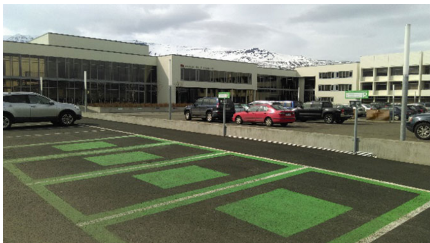
Fig. 21.1 Recharging spots at Akureyri University
