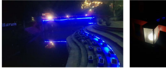
Figure 3. Perimeter illumination at the amphitheater and bridge at Teras Cikapundung in the form blue LED strip light, and bollard.
