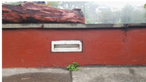
Figure 4. Orientation illumination at stairs at Teras Cikapundung in form of recessed lighting.
