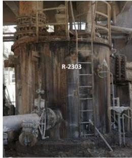
**Gambar 1.3** *Seal Tank Hemihydrate*
